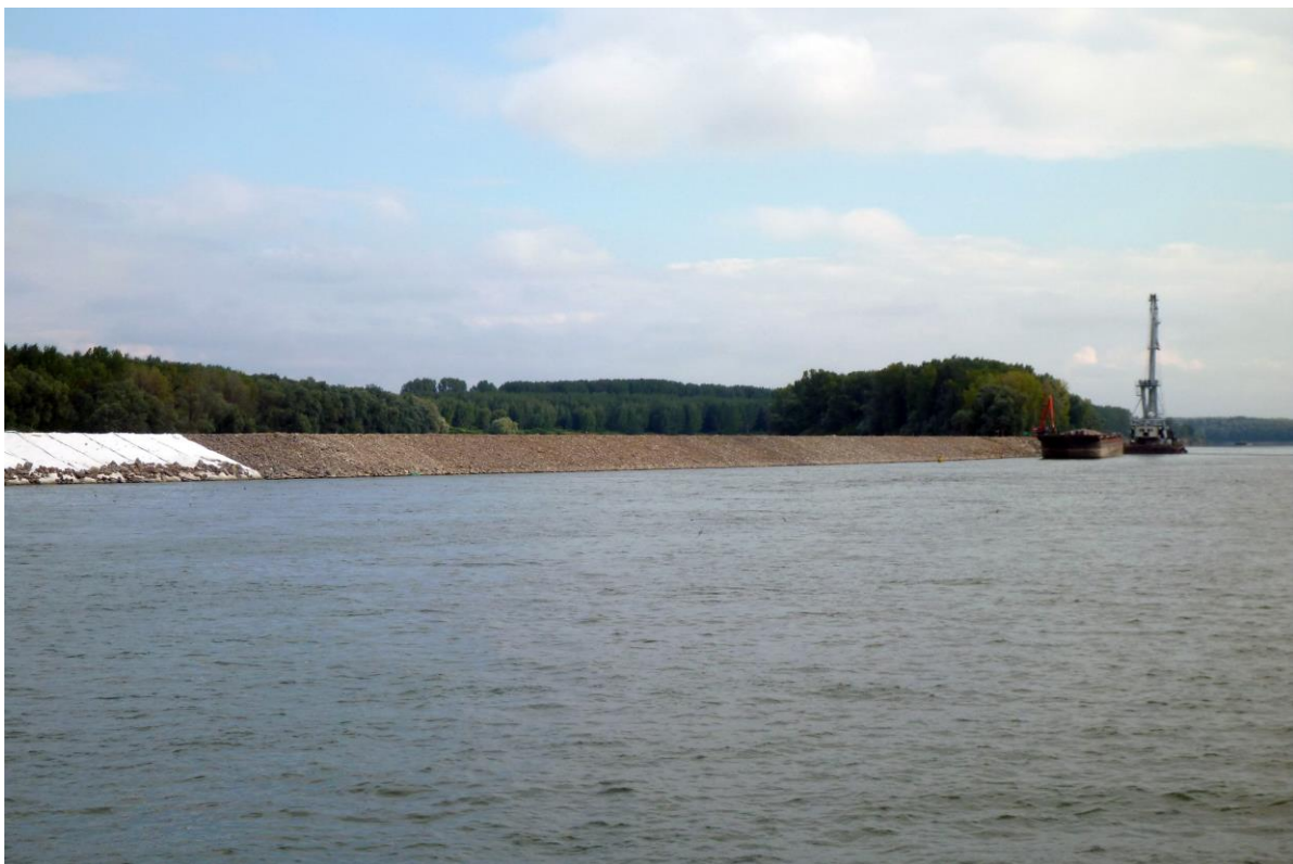
Picture 9: Several fresh bank revetments to stop side erosion and lateral shift are under construction.
