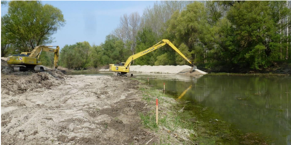
Figure 60: Restoration of side-channel connection along the Slovakian Danube https://broz.sk/obnova-prveho-ramena-klucoveckej-ramennej-sustavy/
